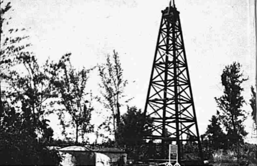
Plate XI Well Number 1, Miri, Fourth Division. First drilled in 1910, this well continues to produce oil. Although production from the Miri oilfield is declining steadily, over 170 wells are still in operation.
