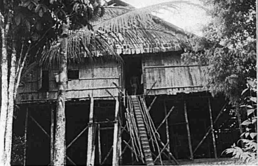
Plate I End view of an Iban longhouse near Sibuan, Third Division, containing twelve 'doors' and housing about seventy people. Over 200 feet long and 70 feet wide it is supported by hardwood posts about 15 feet high.
